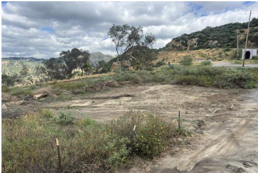
Recent grading activity and vegetation removal on Deck C east end
