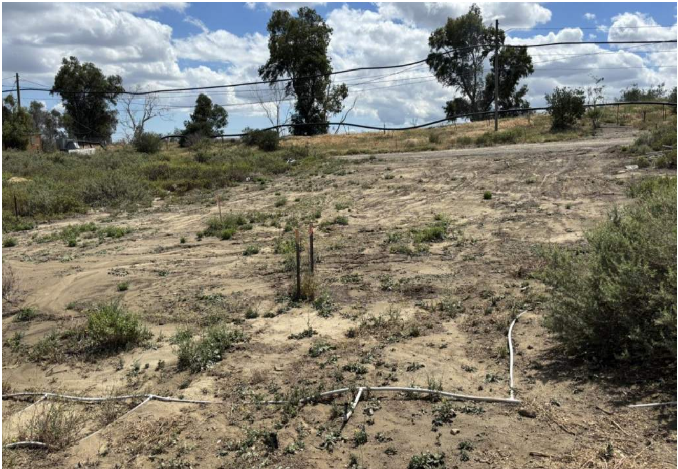
Recent grading activity and vegetation removal on Deck C southwest corner
