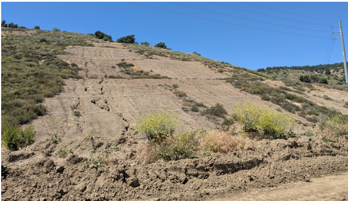
Photograph 2. Facing northwest at the northern portion of the County-Side Sage Mitigation Area where plant growth has been problematic due to poor soil conditions (April 7, 2026)
