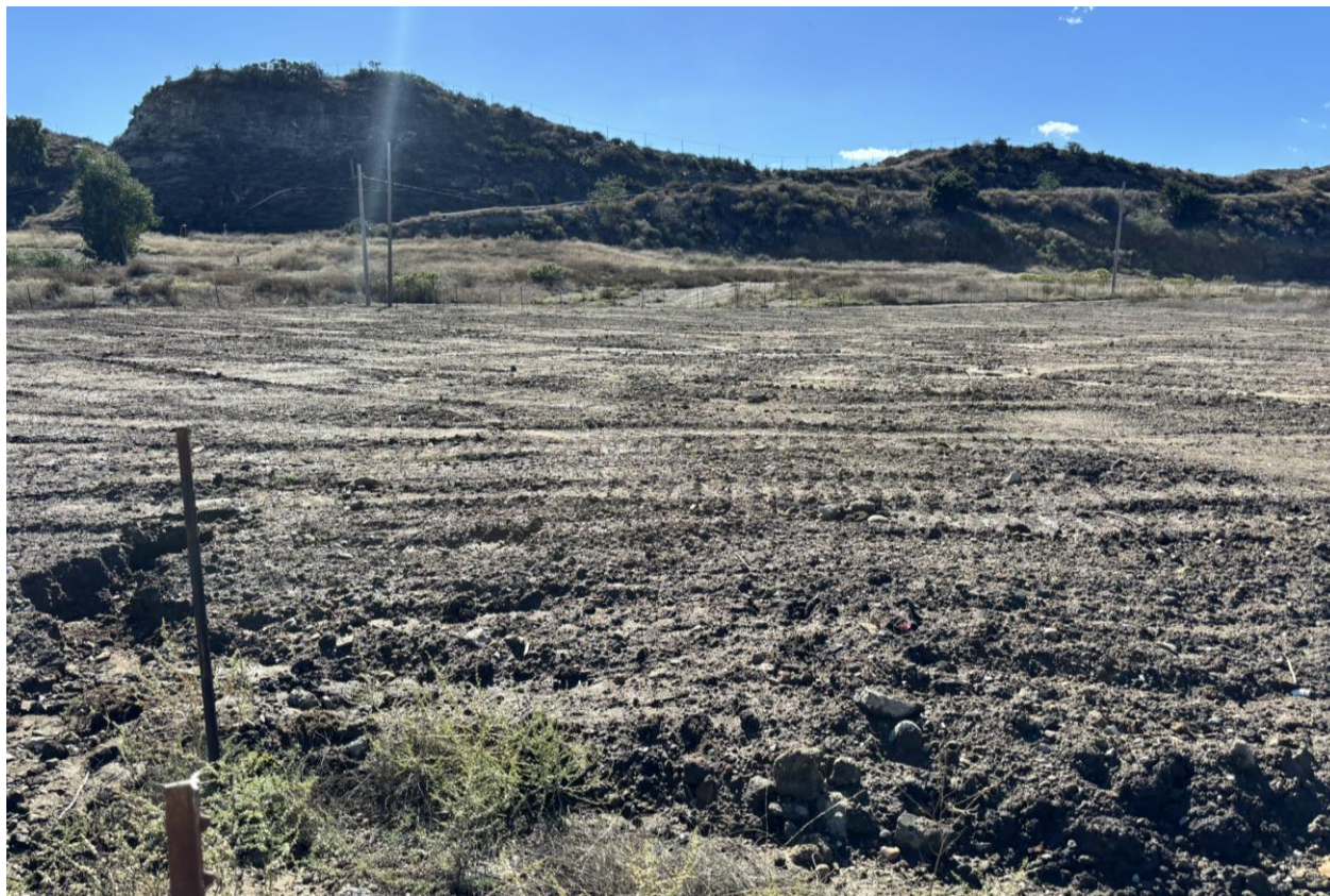
New grading on Deck A to fill in areas where settlement occurred
