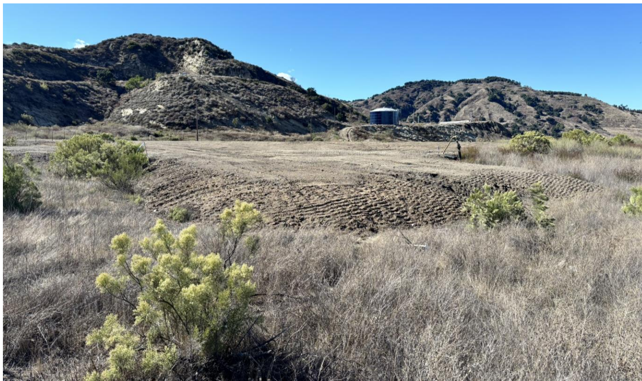
New grading on Deck A to fill in areas where settlement occurred
