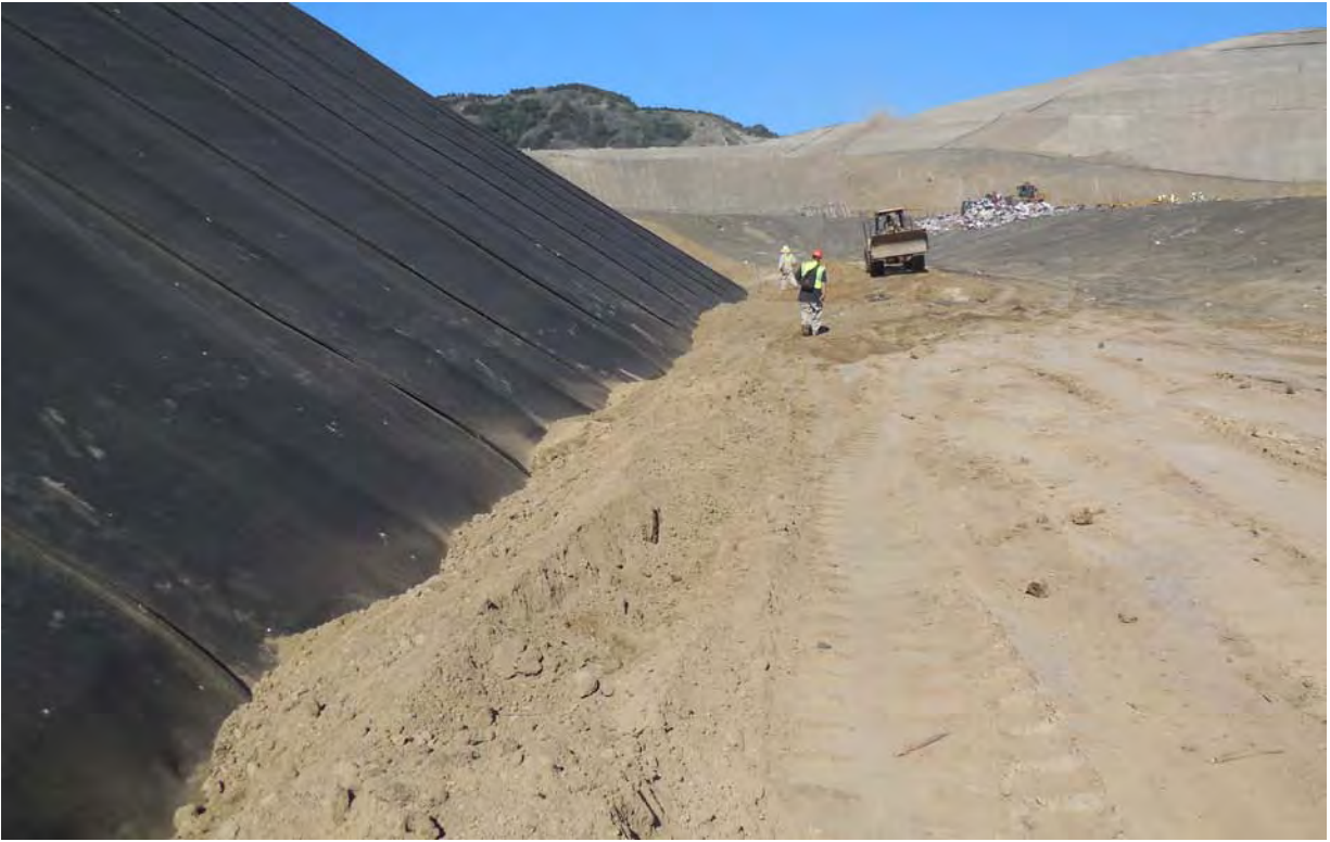
Photo 11 - The protective soil was replaced.
