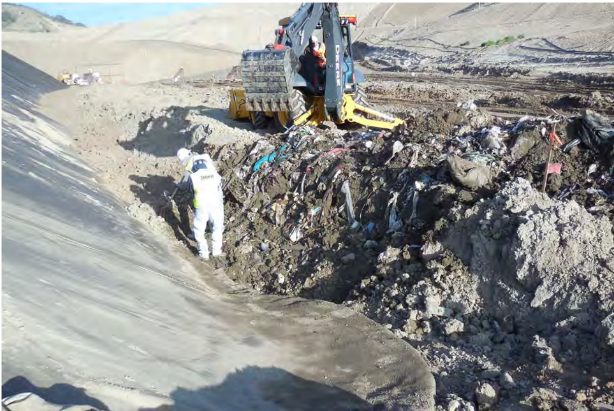
Photo 2 - Refuse and protective cover soil were removed from the affected area.
