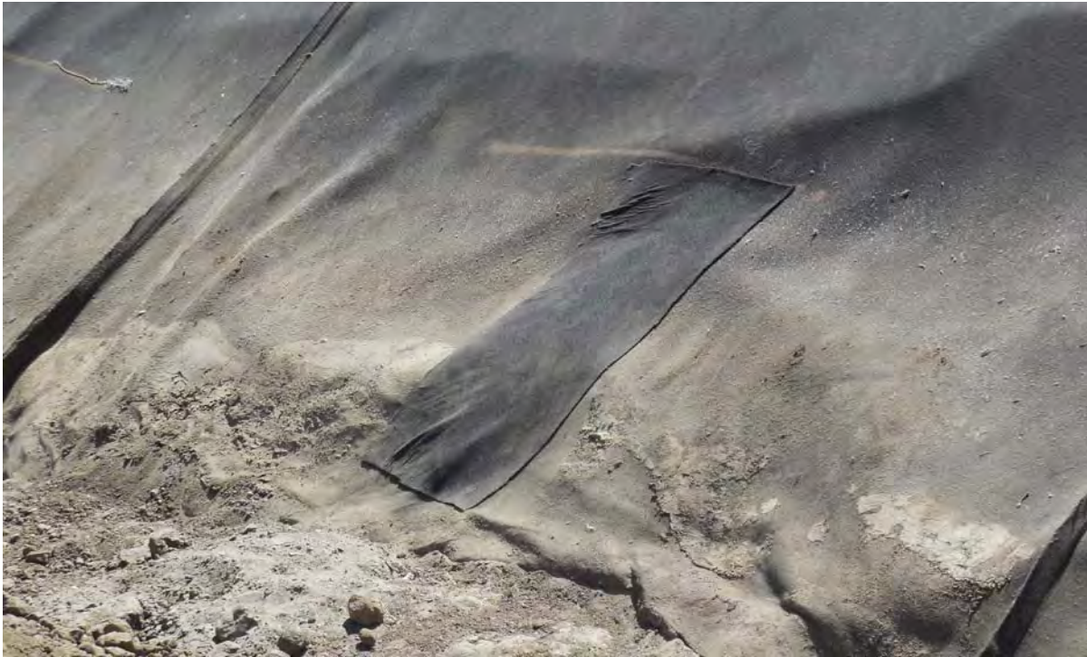
Photo 10 - The geotextile was repaired.
