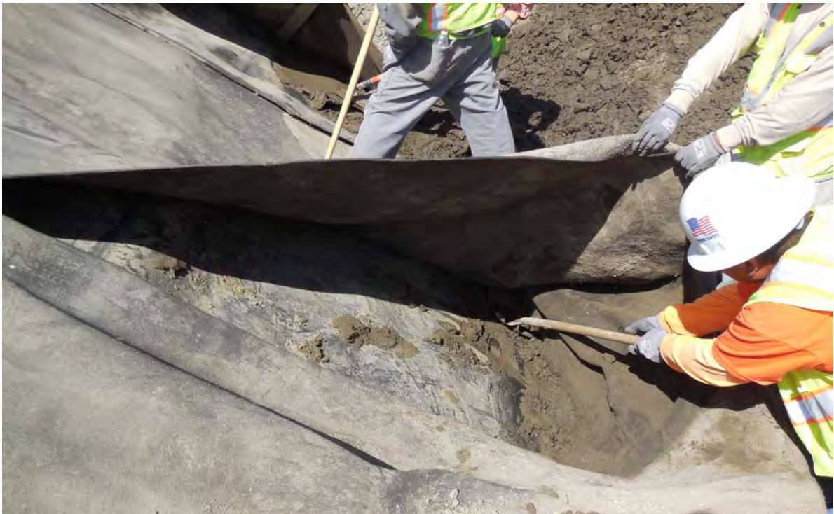
Photo 6 - Fine-grained soils were removed.
