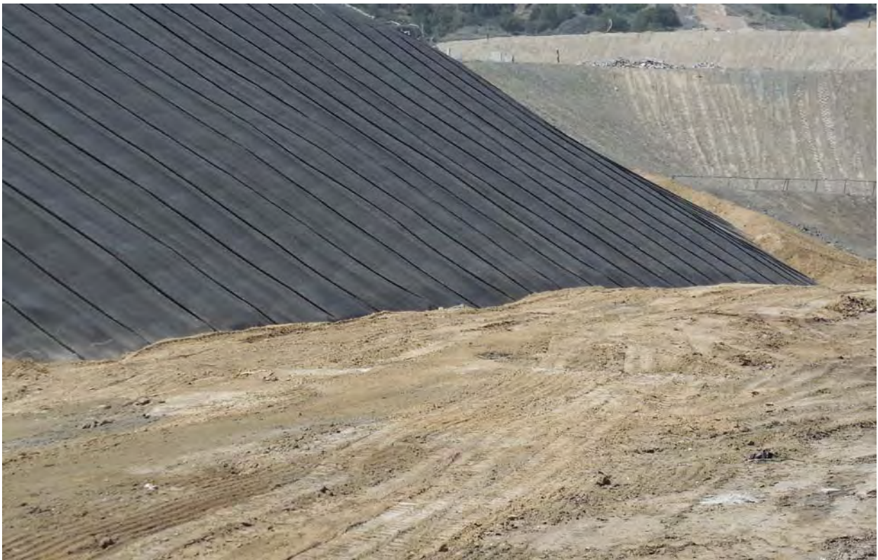
Photo 12 - The protective soil was replaced.
